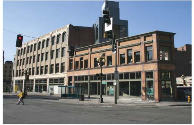
Apex Building from north - after
