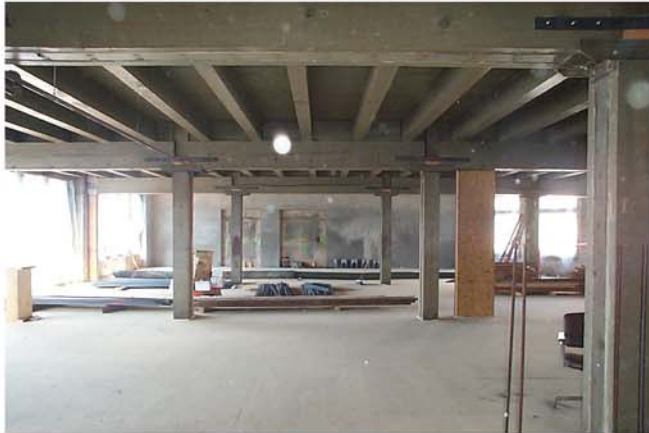
Third Floor Interior - before
