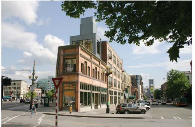
Apex Building from north - after
