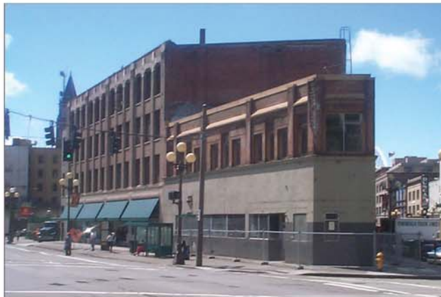
Apex Building - before
