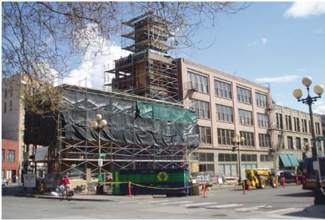
Second Ave. S. - during construction
