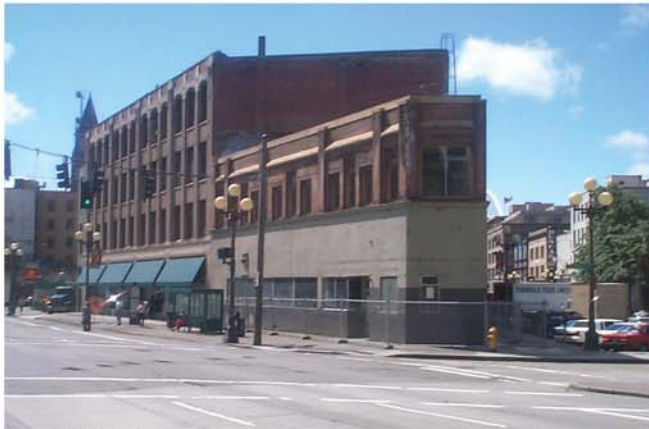
Apex Building from north - before
